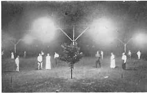
Fig. 1. Golf Practice Course lighted with Mazda lamps and Mazdalux reflectors.
