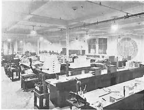
General Illumination with Mazda lamps and Mazdalux reflectors in Bindery of Boot's Printing Works.
